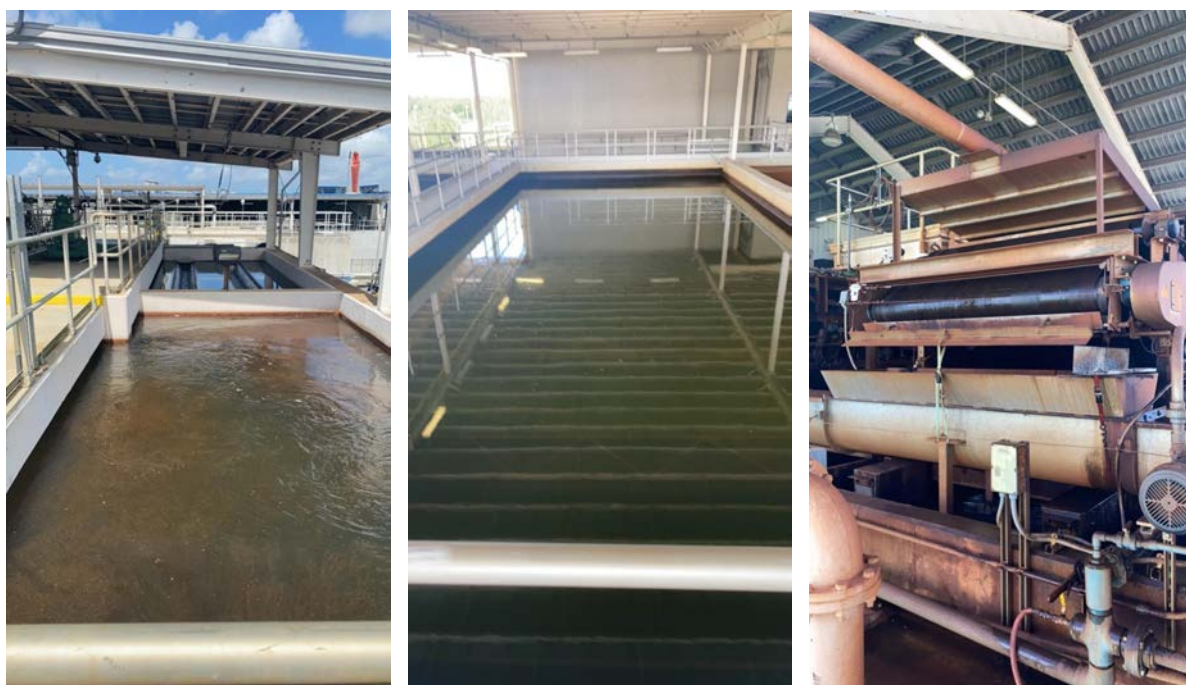
Figure 4-14: Regional SWTP Actiflo, BAF, and Belt Filter Press
