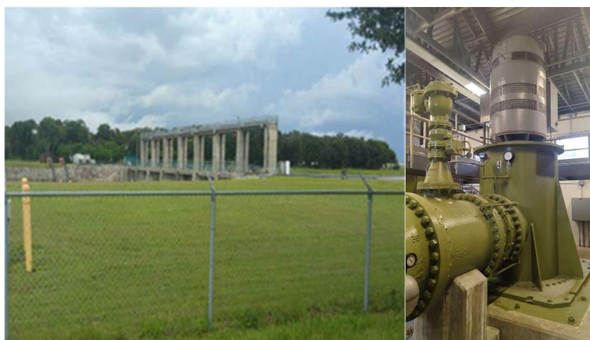
Figure 4-18: Tampa Bypass Canal Intake and Pump Station
