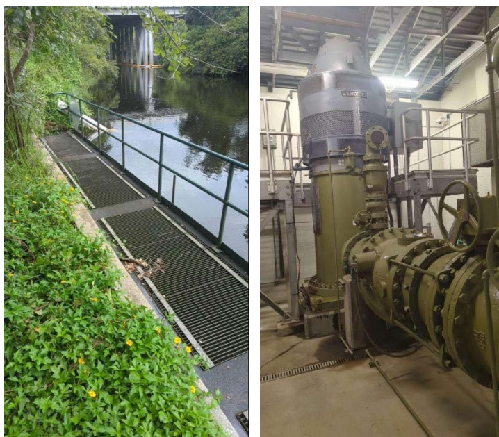
Figure 4-17: Alafia Intake and Pump Station
